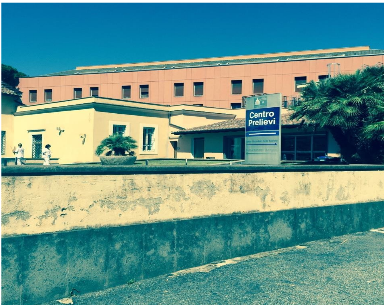
Photo 2: Entrance to TESTING AND SAMPLING CENTRE – Via San Giovanni in Laterano, 155
